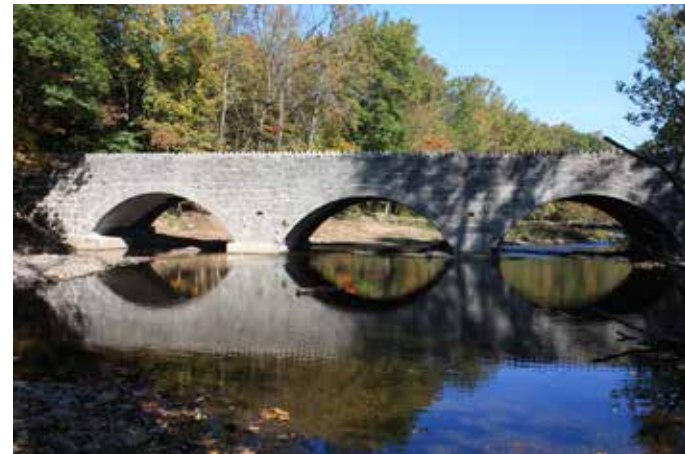
Swamp Creek Road Bridge – North
