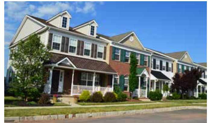
Below: A completed building in Northgate
