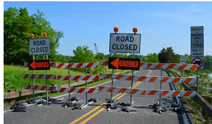
Maintenance of existing roadways and bridges is an ever-present objective
