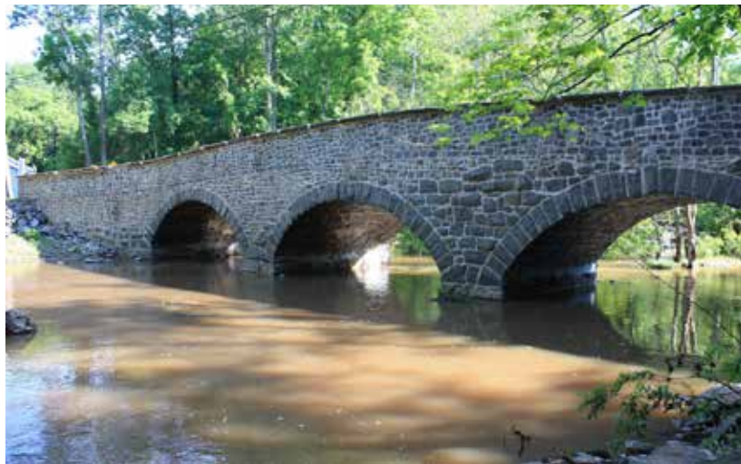
Swamp Creek Road Bridge, a historic resource
