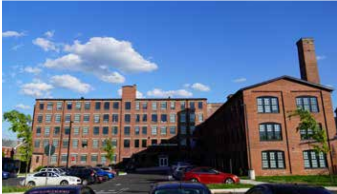
The rehabilitated Boyertown Burial Casket Company
