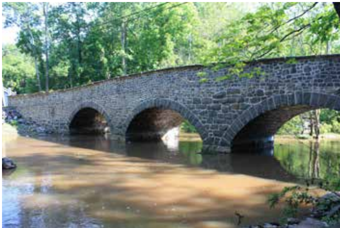
Swamp Creek Road Bridge – South
