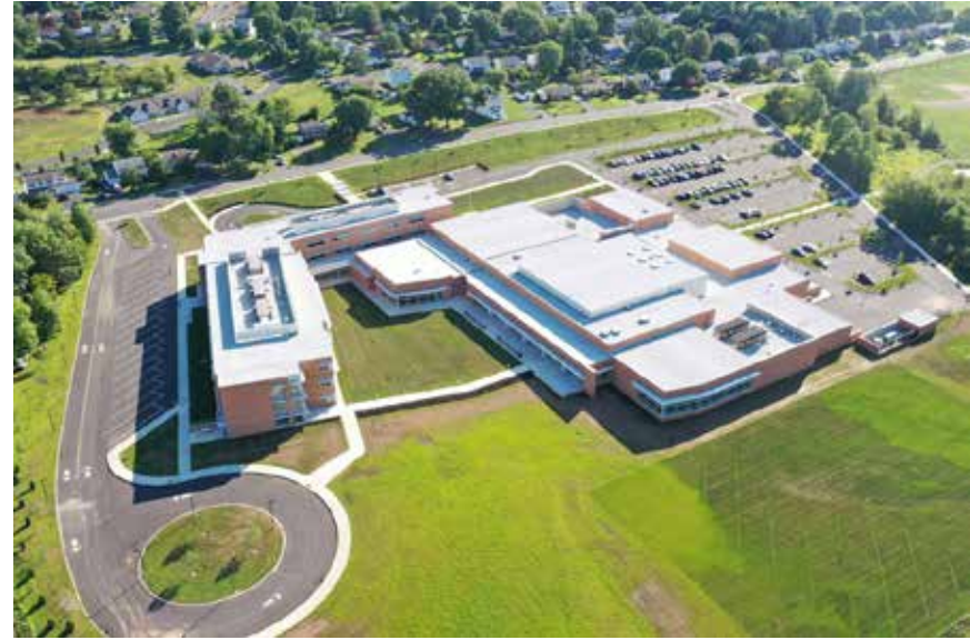
Upper Perkiomen Middle School and High School (Source: Breslin Architects)™
