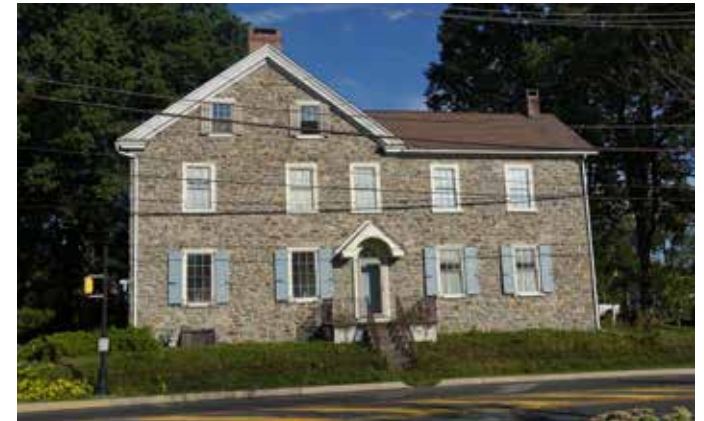
William and Caroline Schall House as viewed from Main Street, 2022
