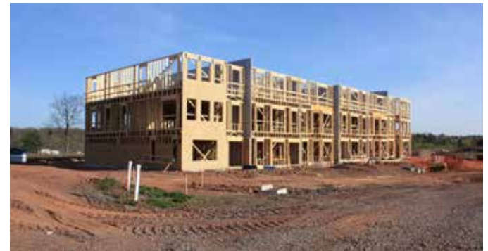
Above: A Northgate building under construction
