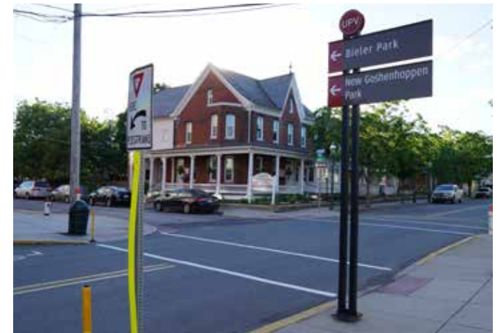
This difficult crossing for pedestrians, near the UPV Chamber of Commerce in East Greenville, includes curb bumpouts, painted crosswalks with signage, detectable warning plates at curb ramps, decorative paving, and pedestrian-operated flags. The flags were recently added as a way to aid pedestrians in getting drivers' attention—an innovative fix!
